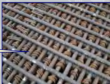
Shear Reinforcement REDUCED
