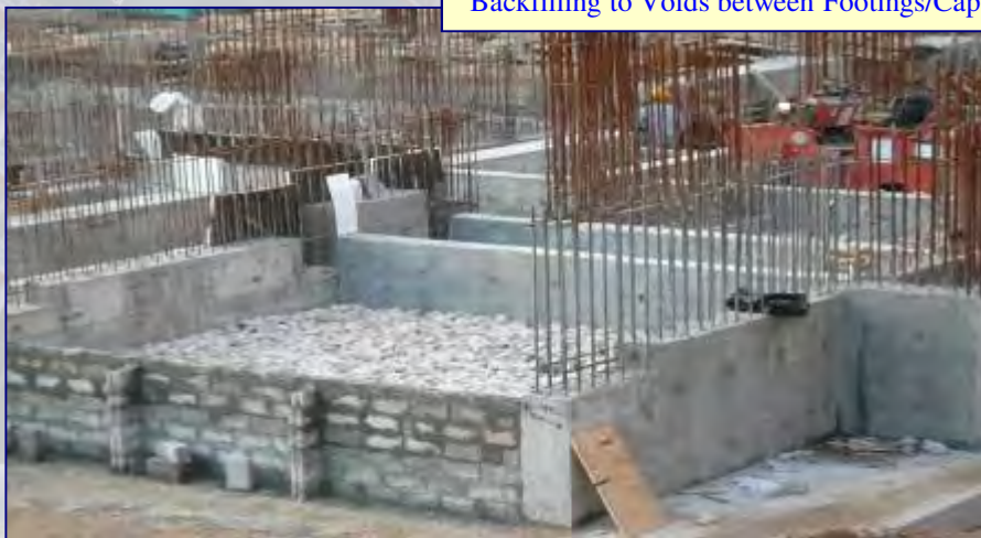
Backfilling to Voids between Footings/Caps and Underside of Suspended Ground Floor Slabs
