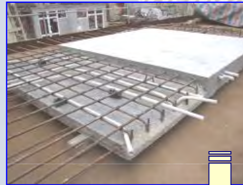
Traditional Semi-precast slab
