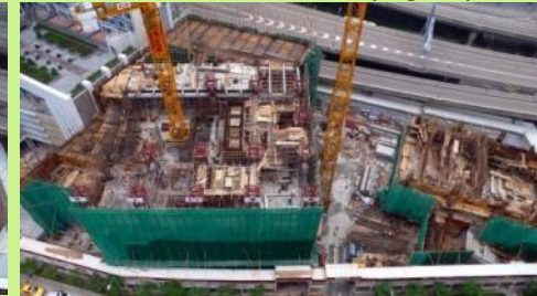
Aerial site progress photos
