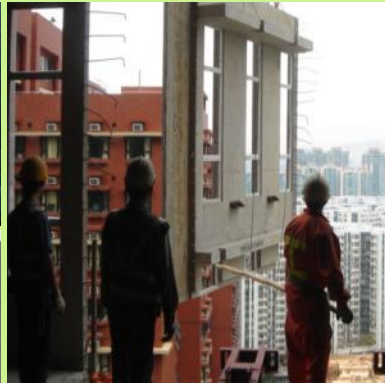
Pre-cast manufacturing & installation
