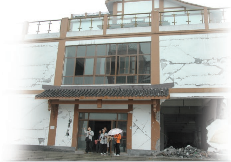
■ 地震對四川建築物的破壞 Quake-damaged buildings in Sichuan
