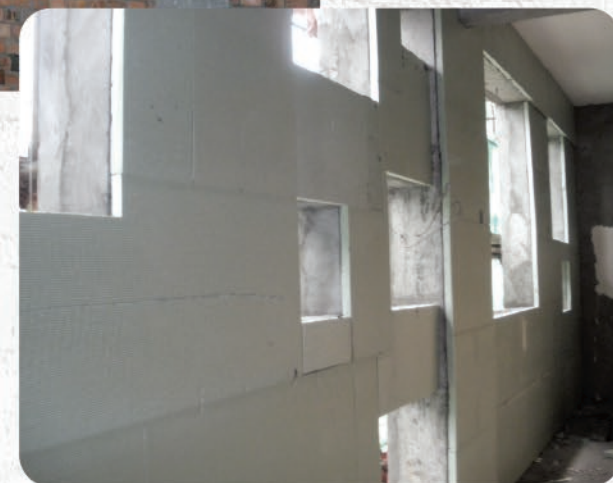
■ 施工中的牆身孔洞 Holes in the wall during construction
