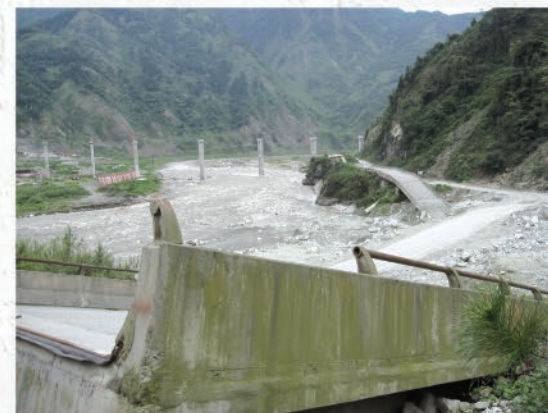
■ 損毀的路橋 A damaged bridge
