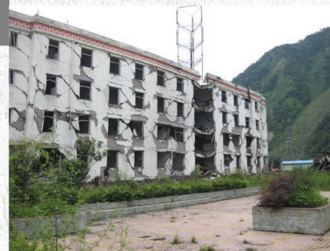
■ 地震中損毀的校舍 School building damaged in the quake
