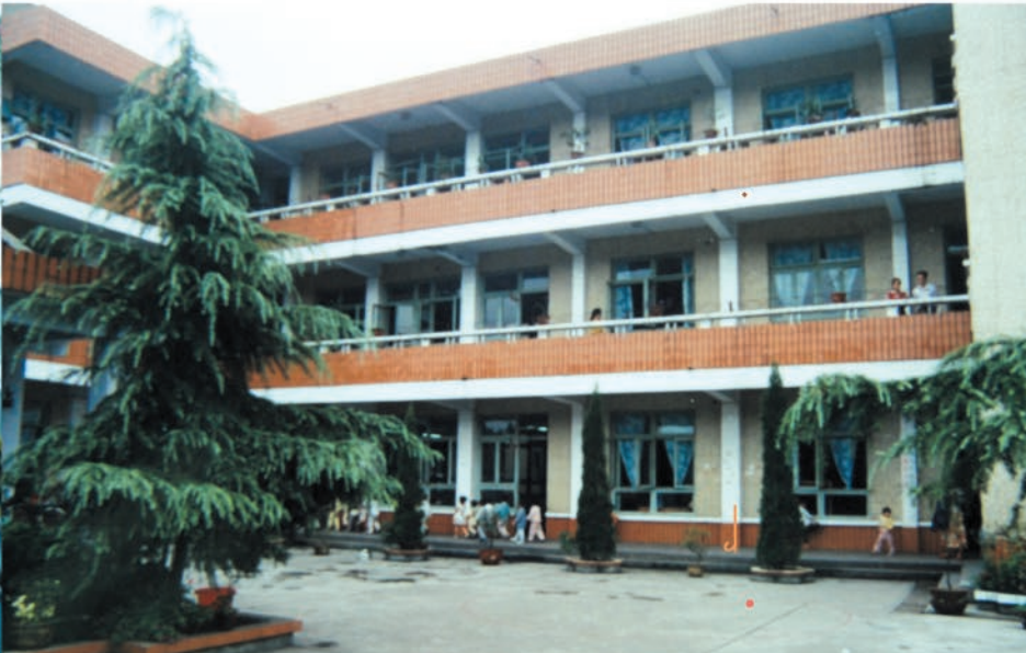
■ 「正東街幼兒園」原貌 Zhengdong Jie Kindergarten before the earthquake
