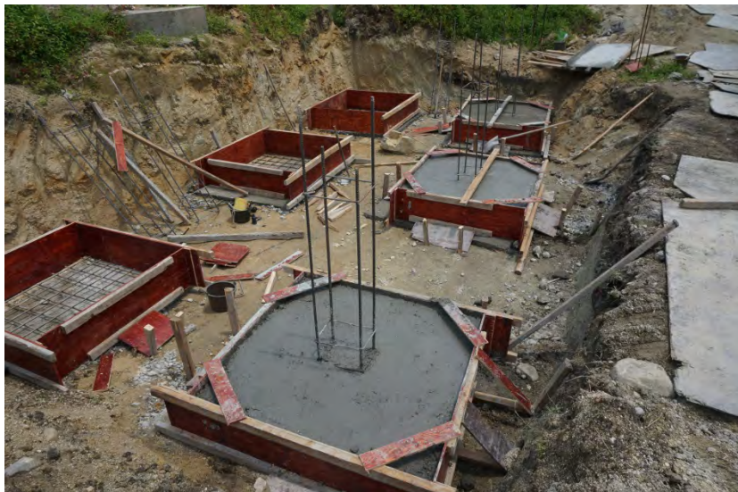
Figure 10 Completion of concreting for footings
