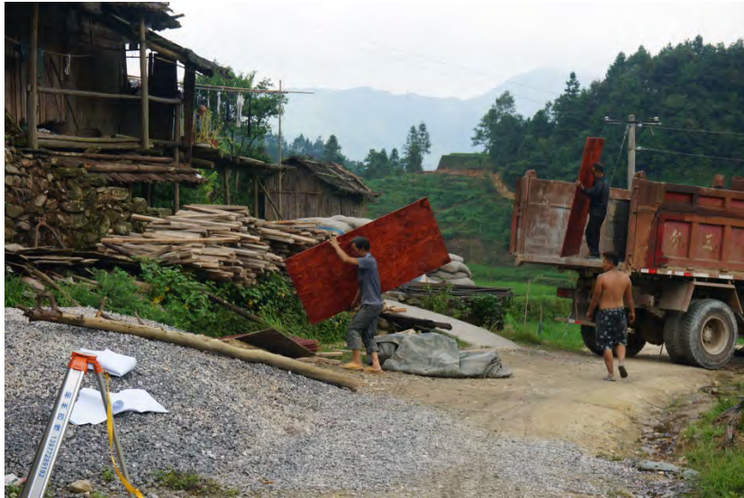
Figure 7 Construction material arrived at Dabao
