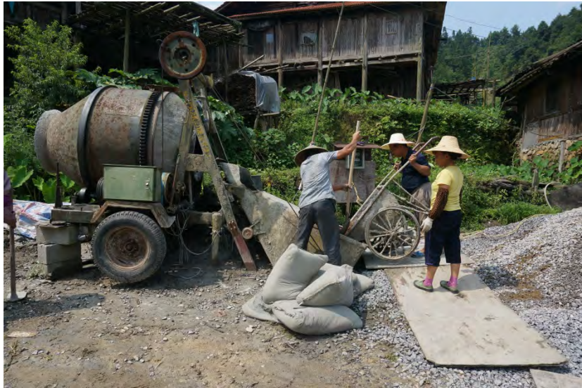
Figure 9 Workers mixing concrete for concreting of footings
