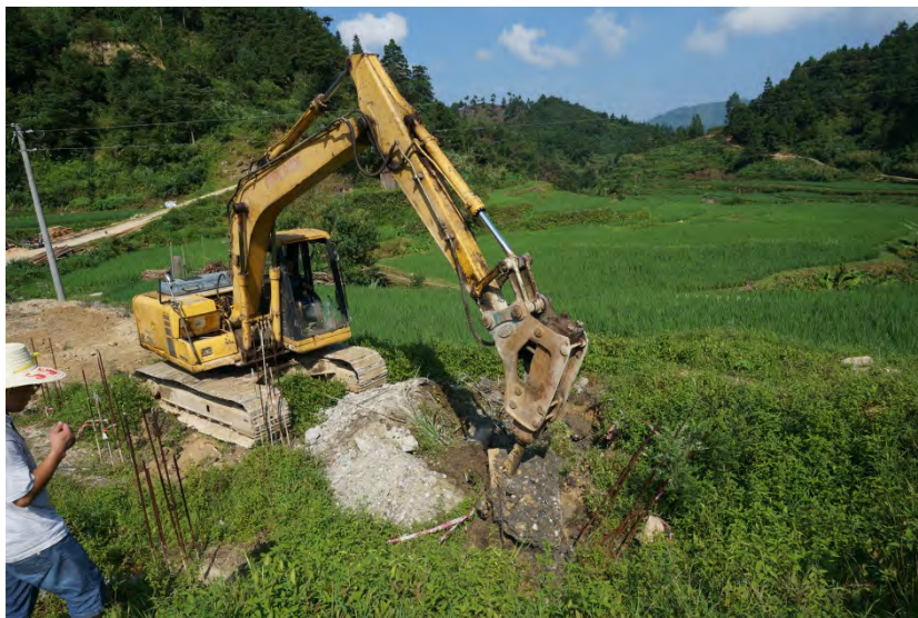
Figure 8 Demolition of wrongly installed footings
