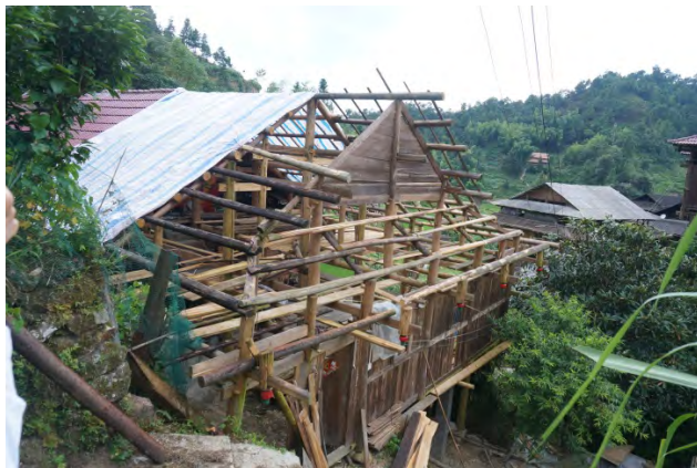
Figure 5 Construction of diaojiao building(吊脚樓)
