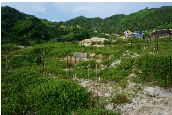
Figure 3 Construction site in Dabao Village, showing the wrongly installed footing, demolished and new footings were re-constructed afterwards.
