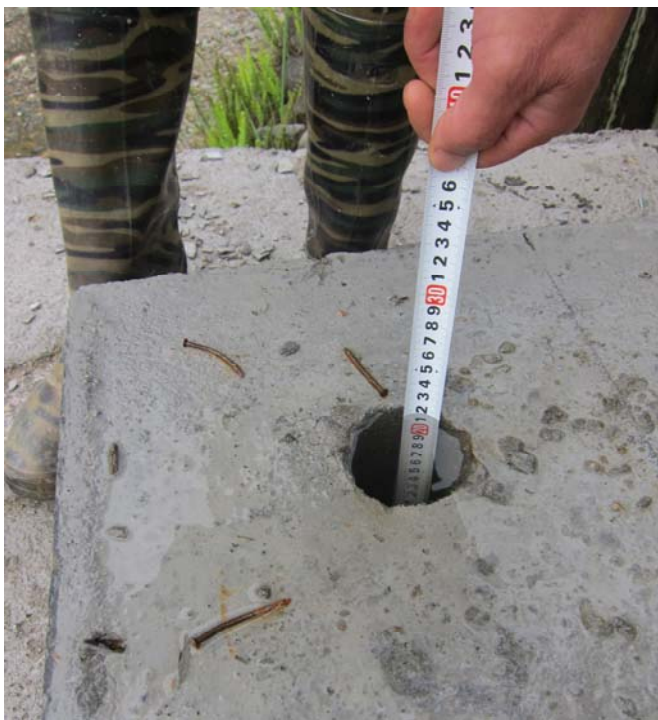
Figure 4 The design depth of these holes should be 300mm but 210mm is recorded.
