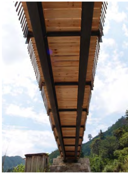
The old and new Yingdong Footbridge.
