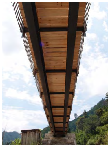
The close-up of the Yingdong Footbridge.
