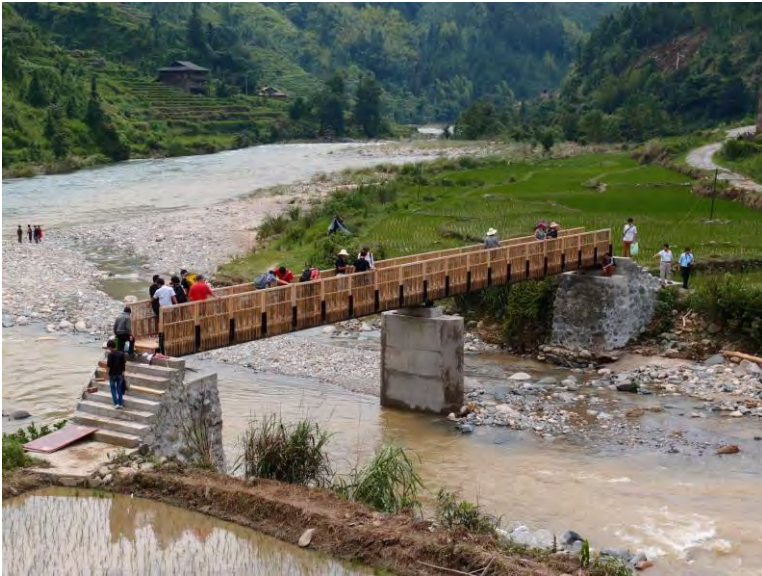
The new Yingdong Footbridge.
