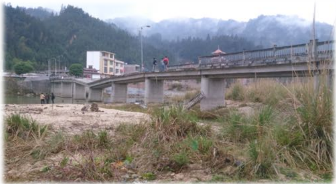
Figure 1 Tengchuen Bridge on 10 th Jan 2017
