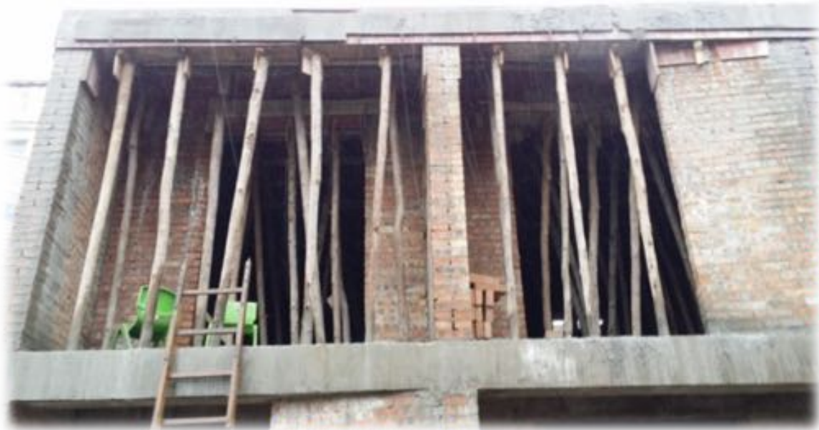
Figure 2 Second Floor of the Teachers' Accommodation of Daping Primary School
