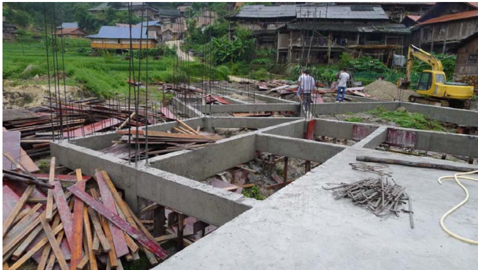
Figure 1 The Dabao building structure as view from the top of the medical room.
