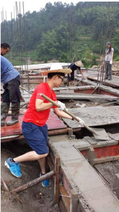
Figure 2 Lau Cheuk Fu, Tony helped in casting concrete to the ground beam.
