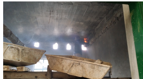
Figure 5. Workers removing nylon bags by burning
