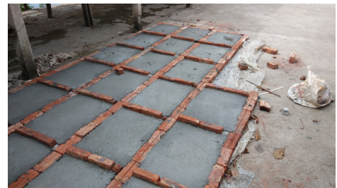
Figure 4. Concreting of channel cover
