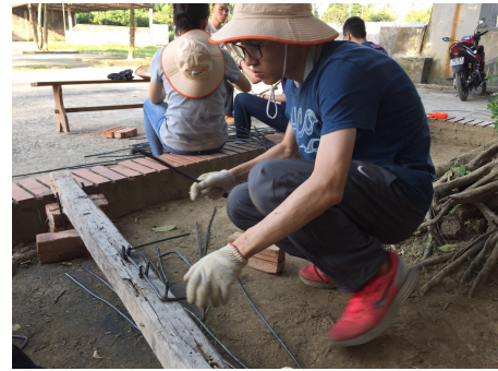
Figure 3. Steel bending by student
