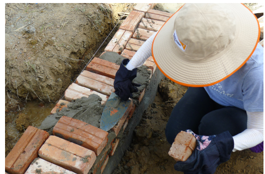
Figure 2. Student constructing brick wall
