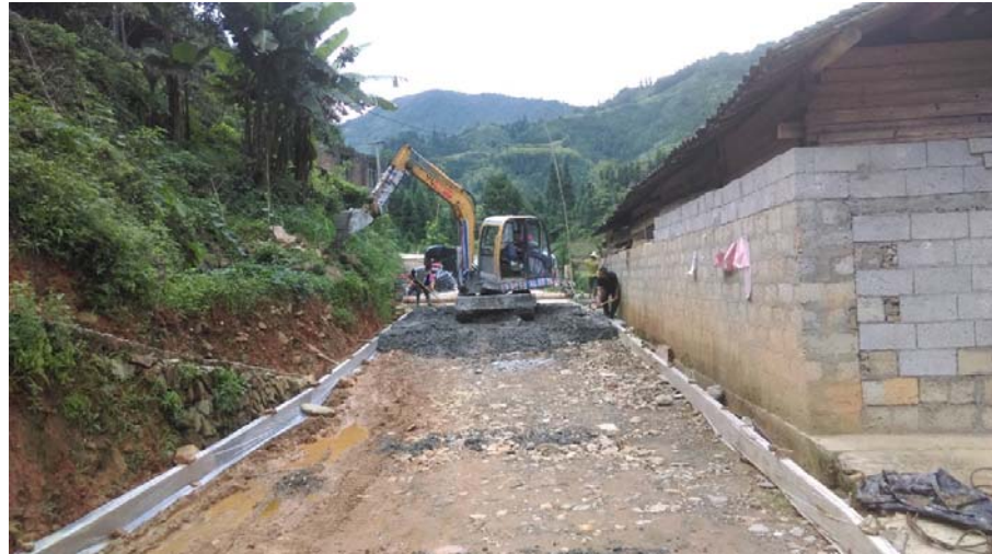
Renovation of the only road to Daping Village
