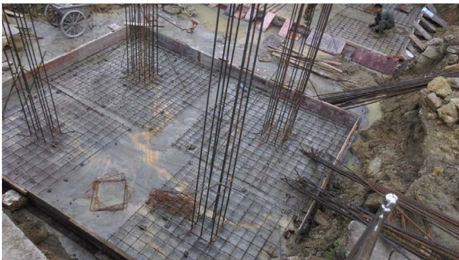
Construction site in Tonglian
