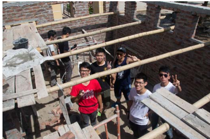
Fig. 3: Brick wall construction.
