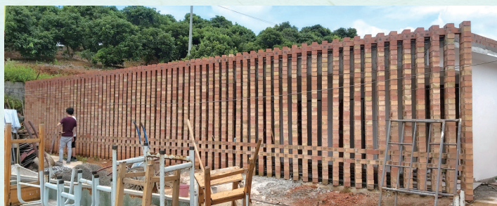
An innovative design of façade wall to allow natural lighting and ventilation.
