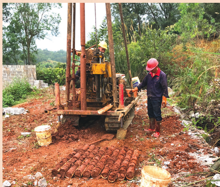
Ground investigation for the proposed composite building.
