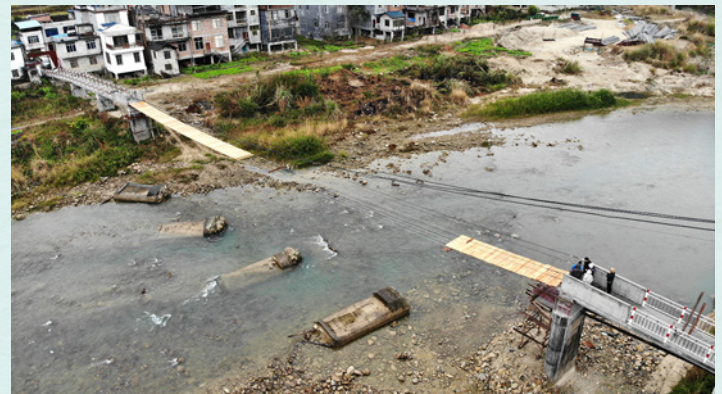
Laying a wooden deck on the steel cables for Wangdong Footbridge.
