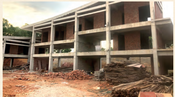
The reinforced concrete frame of the Composite Building was successfully completed in July.
