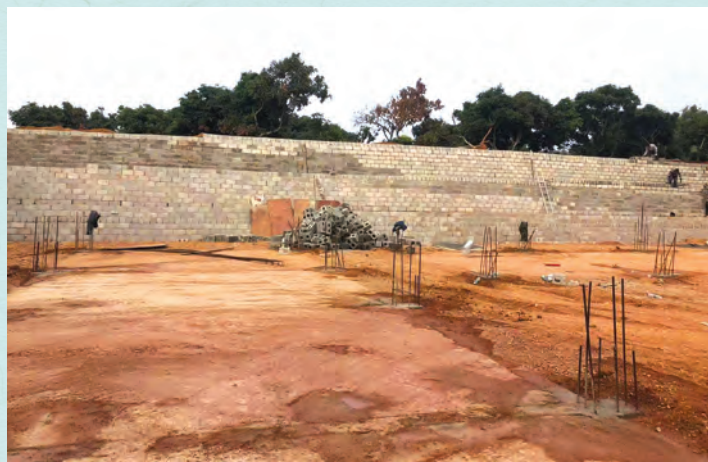
A retaining wall was constructed to support the slope next to the Composite Building.
