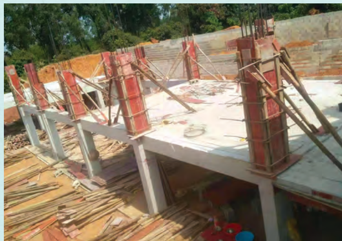
The Composite Building was building in progress, the reinforced concrete frame is anticipated to be completed by this June.
