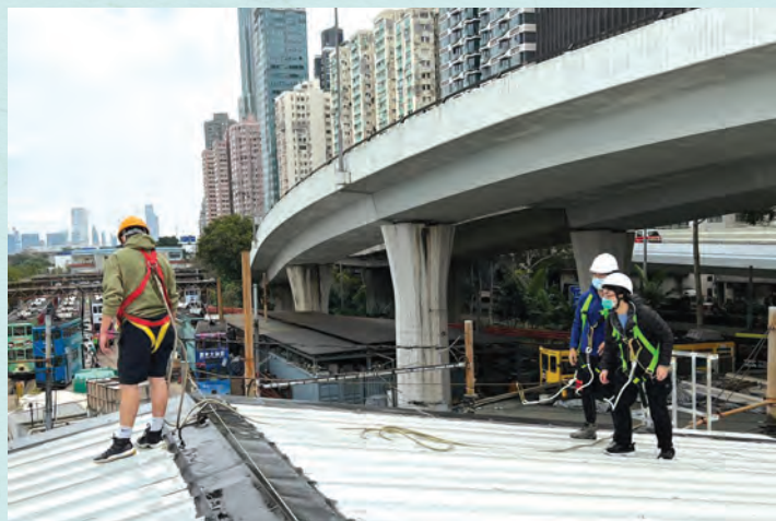
Roof maintenance work was completed, and students participated in the water sprayed test at the roof area to verify the quality of workmanship.
