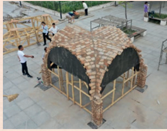
Students created prototypes and gained practical on-site experience in brickwork.
