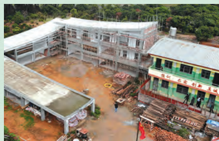
The reinforced concrete frame of the Composite Building had been completed.
