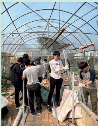
Our students were building planting trays and constructing a siphon system.
