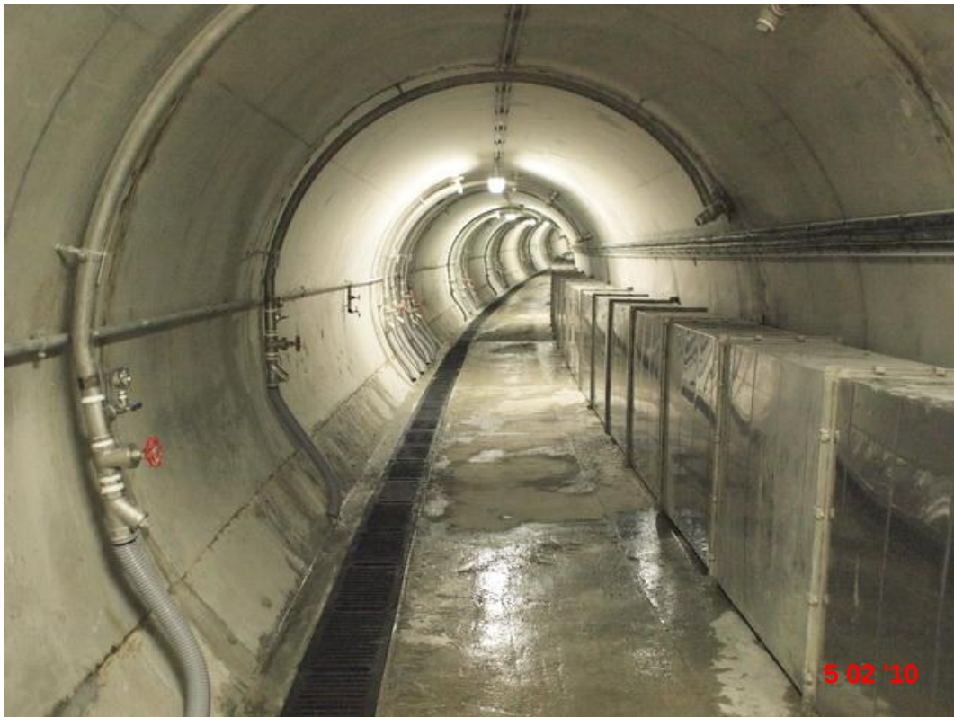
Fig. 8 Sub-vertical drains installed inside tunnel with permanent concrete lining
