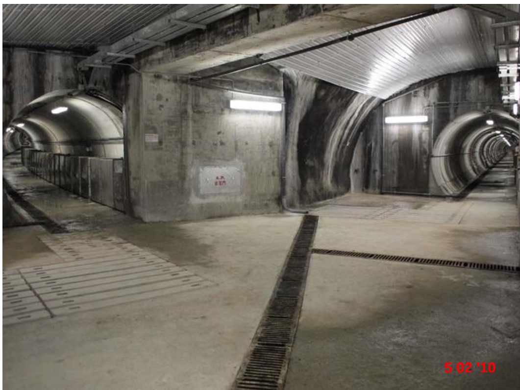
Fig. 9 Drainage tunnels - high tunnel on the left and low tunnel on the right.
