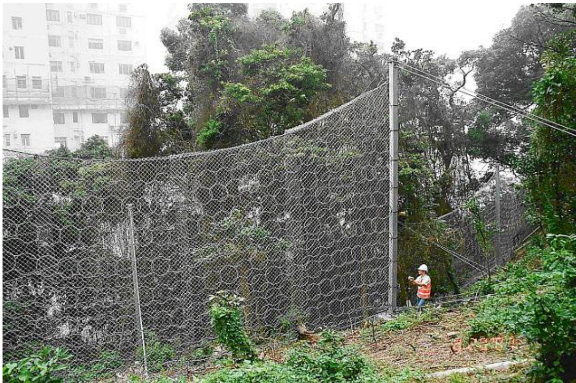
Fig. 7 Flexible barrier as part of mitigation works for shallow landslides
