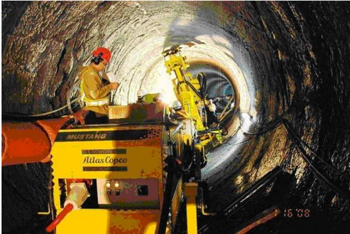
Fig. 6 Installation of sub-vertical drains
