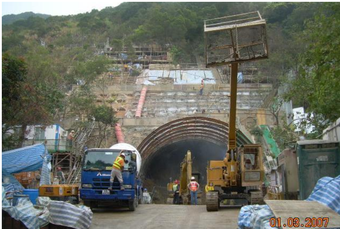
Fig. 6 Excavation of tunnel portal
