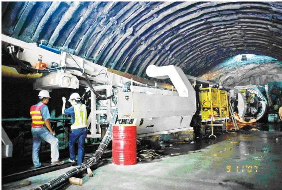
Fig. 5 TBM being assembled on site
