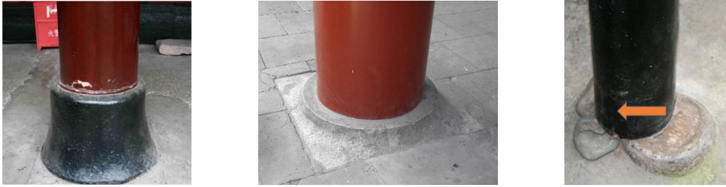
(a) Type 1(before slipping) (b) Type 2(before slipping) (c) Type 3 (After slipping) Fig.5 Typical Connection method between column foot and foundation
