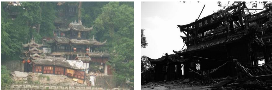
Fig.1 Destroyed cultural heritage buildings in the Wenchuan earthquake
