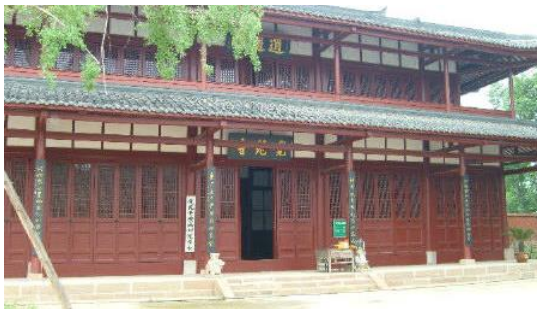
Fig.3 Chinese traditional wooden structure
