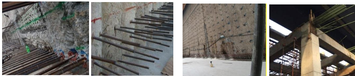
a) Application of post-installed rebars to replace misaligned couplers of basement diaphragm walls (left) and missing starter bars of concrete bored piles (right)
