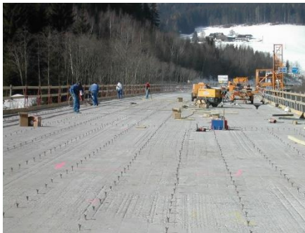
a) Bridge deck strengthening
