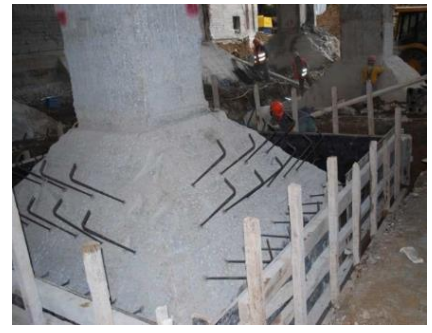
c) Foundation strengthening
