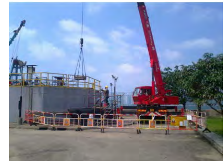
Removal of scum from Drop Shaft at Chai Wan Preliminary Treatment Works
