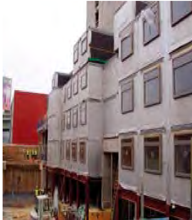
Installation of module on steel podium
