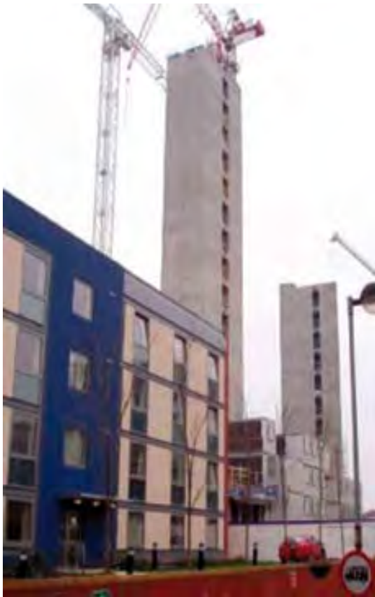
Modules attached to concrete core
