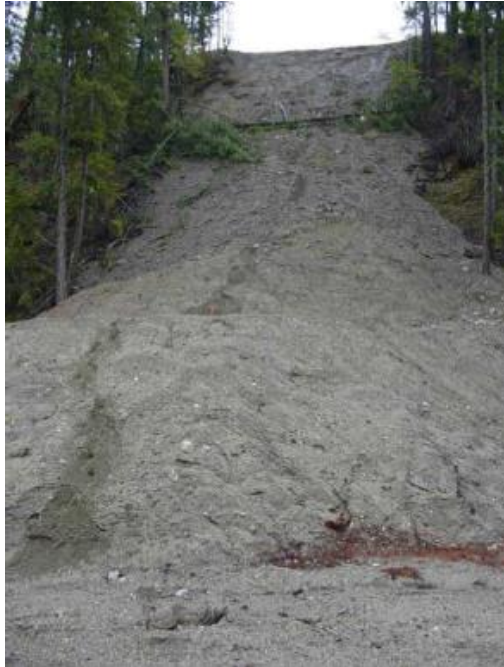
Surficial erosion due to heavy runoff
