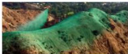
Figure 1. Aerial Hydroseeding ( http://www.arkisomarciviana.com/hydroseeding.php )
