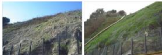
Figure 2. Combined rockfall nets with hydroseeding in Orvieto (Italy): On the left: vegetation after one month; on the right: vegetation established after 8 months (source Prati Armati: http://www.pratiarmati.it/ ).
