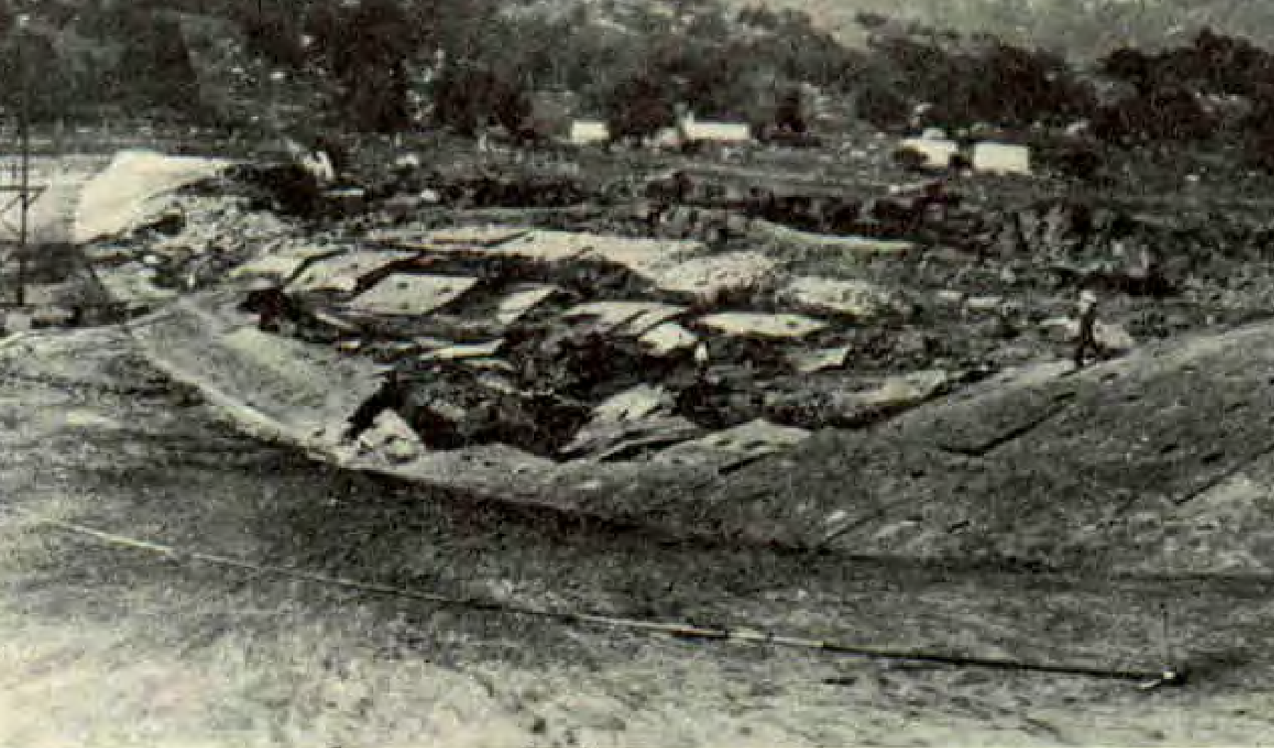
Fig. 10.60. Failure of Sheffield Dam during Santa Barbara earthquake (1925)
