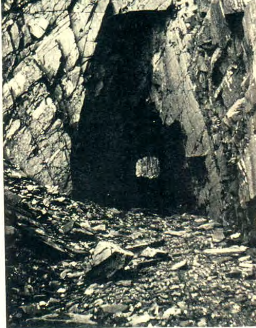
Figure 1 : A tunnel in slate showing the influence of structural discontinuities upon excavation stability.
