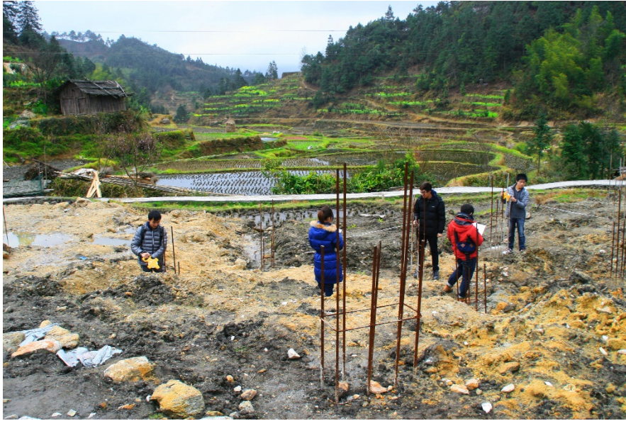
Figure 2: Students checking the completed foundation of Dabao Community and Cultural Centre
