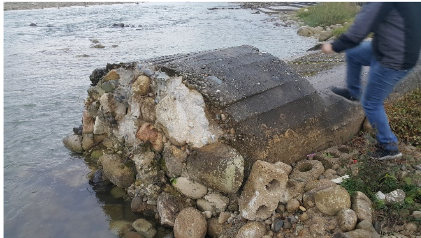
Figure 3 Collapsed old bridge Pier
