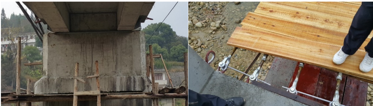
Figure 2a and 2b The cables wrapping around the pier and the structure of the pin joint
