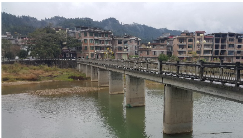
Figure 4 The Tengcun Bridge after righting
