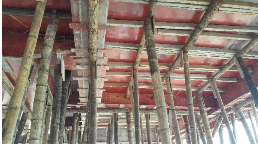
Figure 5 The falseworks and formworks on-site
