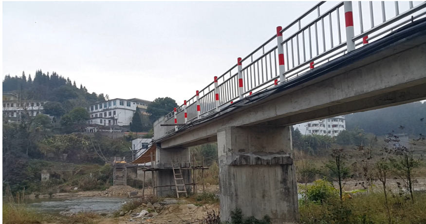
Figure 1 The Construction site of the suspension footbridge
