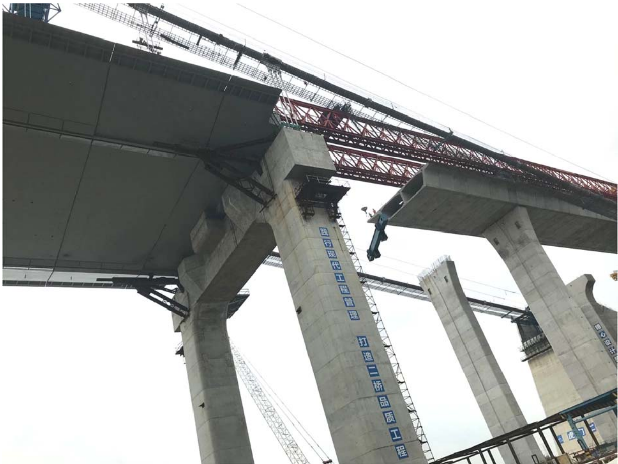
Fig.1 Humen Second Bridge
