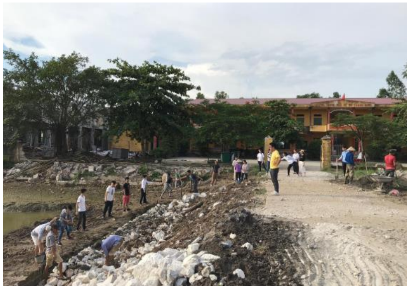
Fig.1 Doing construction work
